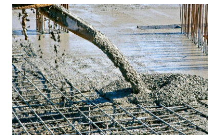
Slab Casting
