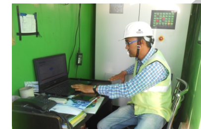
Mixing Control Room
